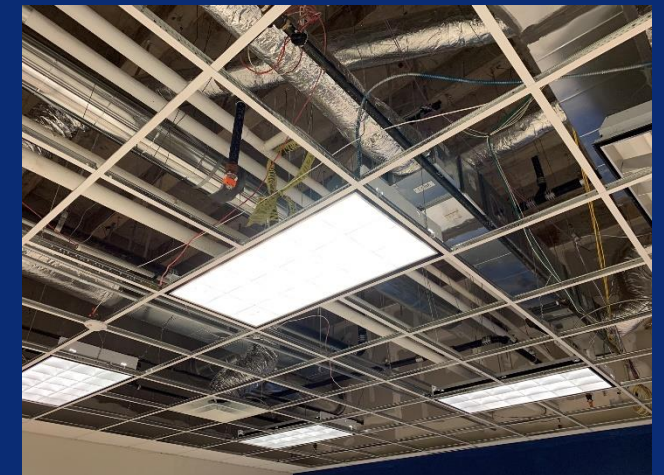
Overhead in Area K Classroom
