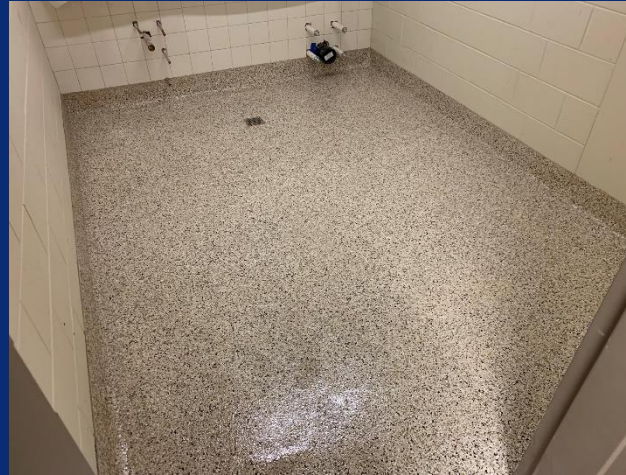
Epoxy Flooring in Area F Staff Restroom
