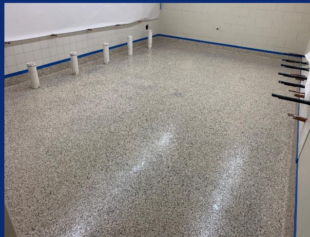
Epoxy Flooring in Area F Restroom
